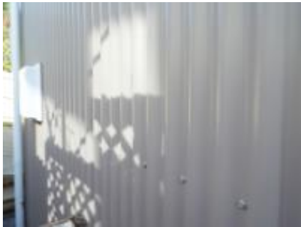
exterior appears well painted
