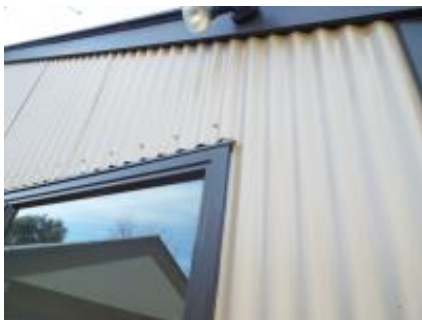
good flashing detail
