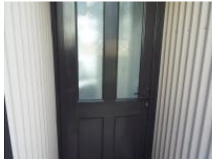
joinery in good working order
