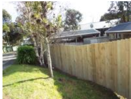
new fence noted
