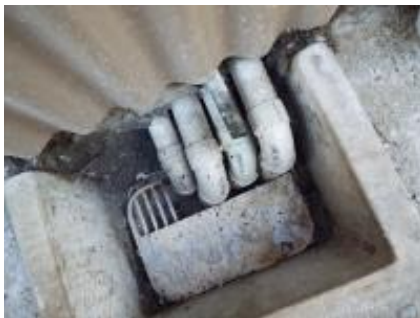
drain clean at the time of inspection
