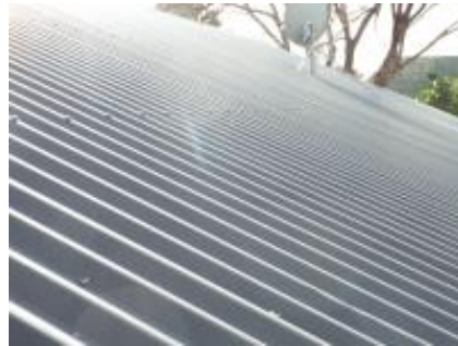
roof appears in good order
