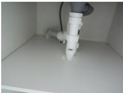
plumbing fine at the time of inspection
