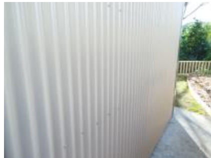
all fine at the time of inspection
